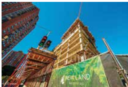
WORLD'S TALLEST HYBRID MASS TIMBER BUILDING, MILWAUKEE. COURTESY OF C. D. SMITH CONSTRUCTION
